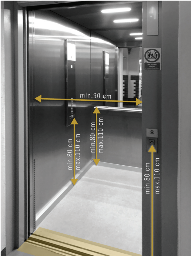
Fig. 2. Elevator in the E-1 building at the Faculty of Architecture of the Wrocław University of Science and Technology with the marking of elements adapted to the disabled
