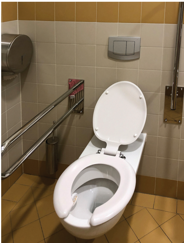
Fig. 6. Toilet for disabled people in building E-5 at the Faculty of Architecture of the Wrocław University of Science and Technology
