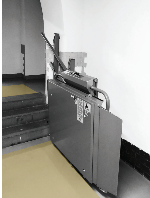
Fig. 3. Side stairlift in the E-1 building at the Faculty of Architecture of the Wrocław University of Science and Technology with the significant manoeuvring space next to the lift marked
