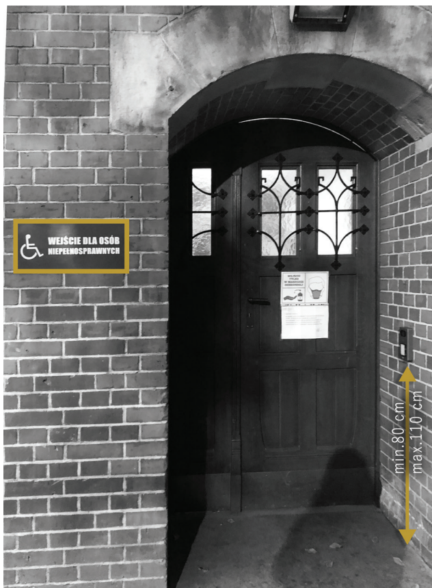
Fig. 1. Entrance to the E-1 building at the Faculty of Architecture of the Wrocław University of Science and Technology, marked with elements adapted to the disabled
